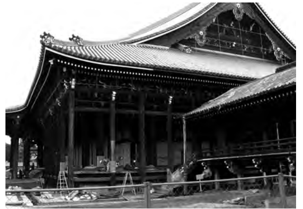
THE GOEIDO (MAIN HALL) IS CURRENTLY BEING RENOVATED.
