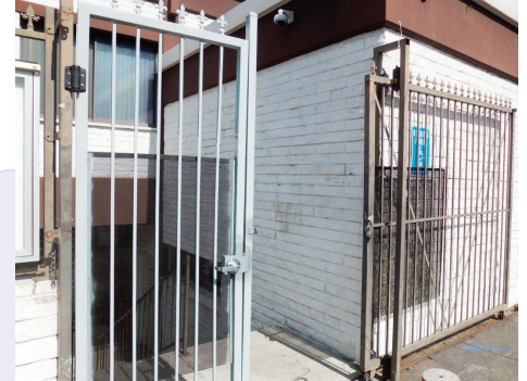
Repaired iron gate
