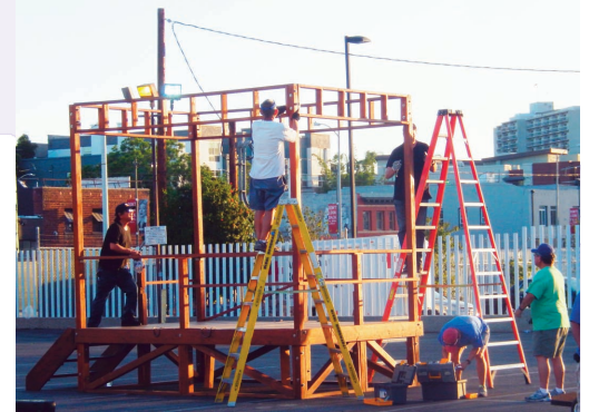
Obon: Dismantling of the yagura
