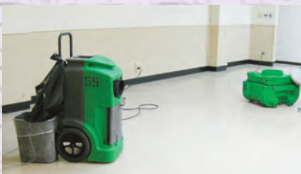
Fans, de-humifiers, and air filters were running throughout the water-damaged areas.
